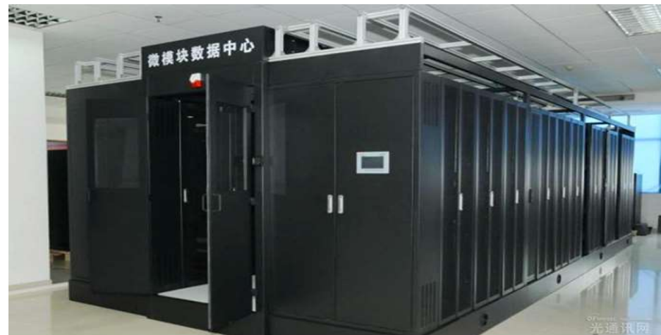
Modular type data center
